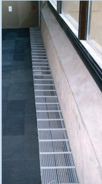
Perimeter Trough for heating and cooling
